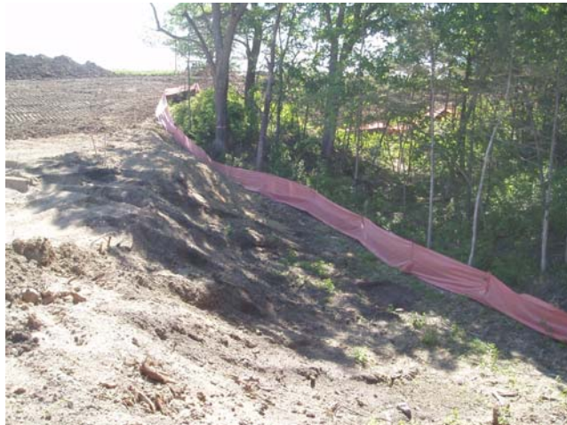
Above: Tree protection fence providing construction limits for grading (2006).
