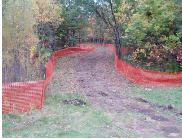
Above: Tree protection fence installed to protect trees along a driveway (2006).
